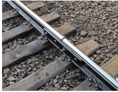
Rail junction at the Beskyd station of the Lviv railway in Ukraine. Photo by Helgi. Shared under a Creative Commons license.
