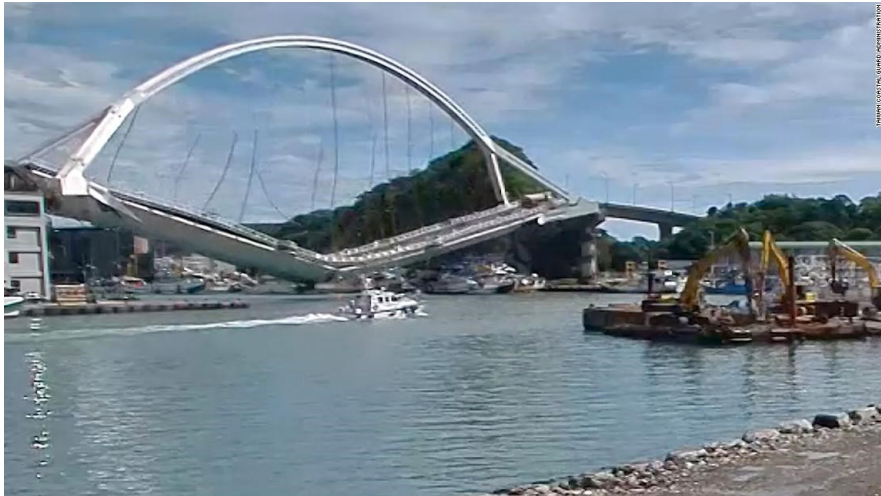
Nanfang'ao Bridge (Taiwan) collapse in 2019. Photo from the Taiwan Coastal Guard Administration.
